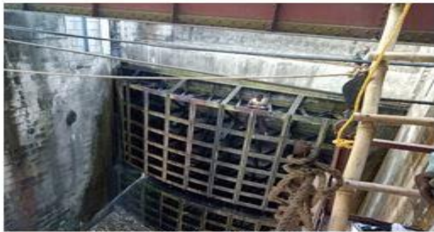
DAM GATES ADJACENT TO THE BRIDGE
