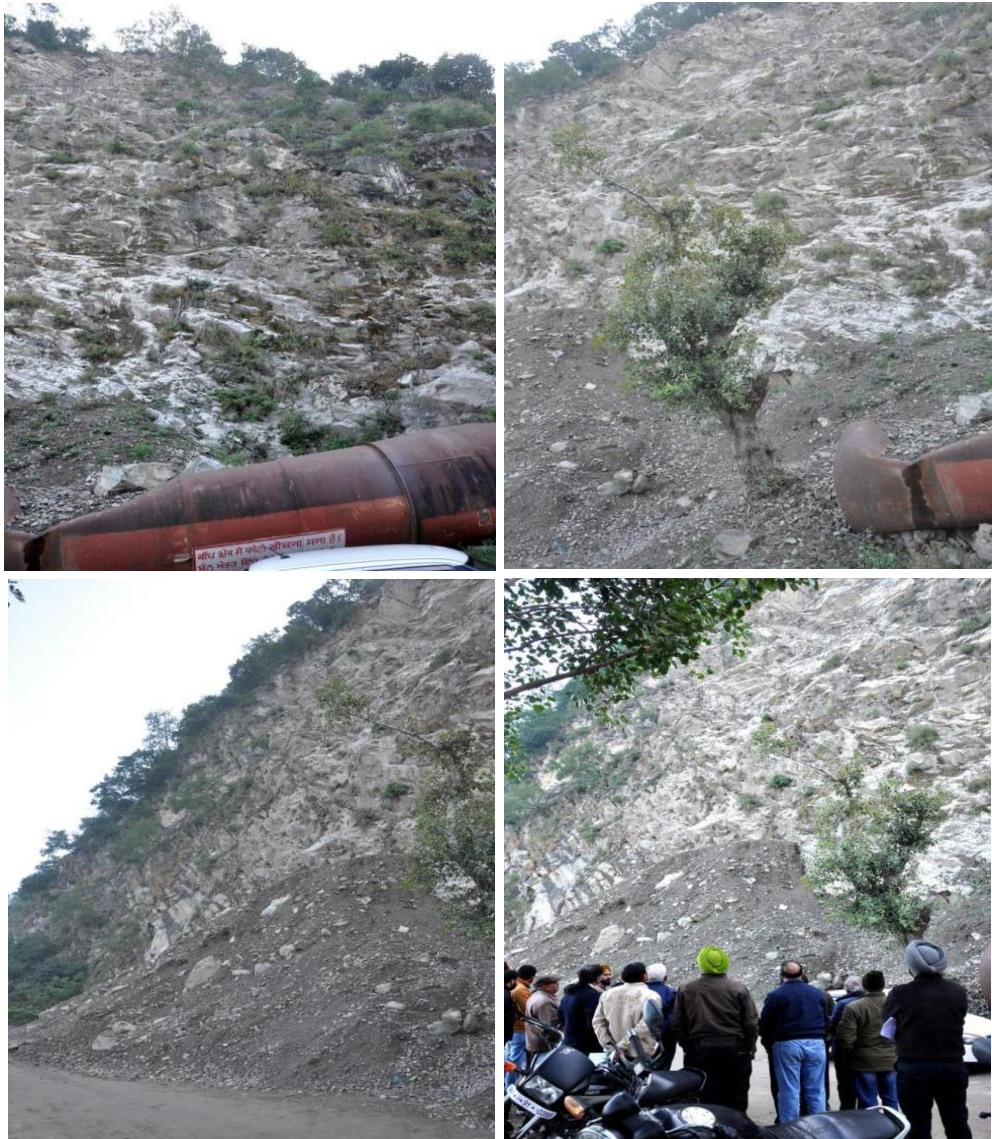
Active Landslide Near Left Abutment on Reservoir Rim
