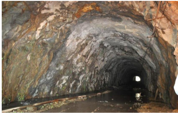
Highway Tunnel near Right Abutment
