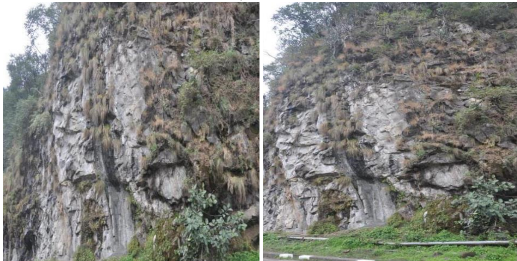
Disposition of Rock Joints near Left Bank Power House Road
